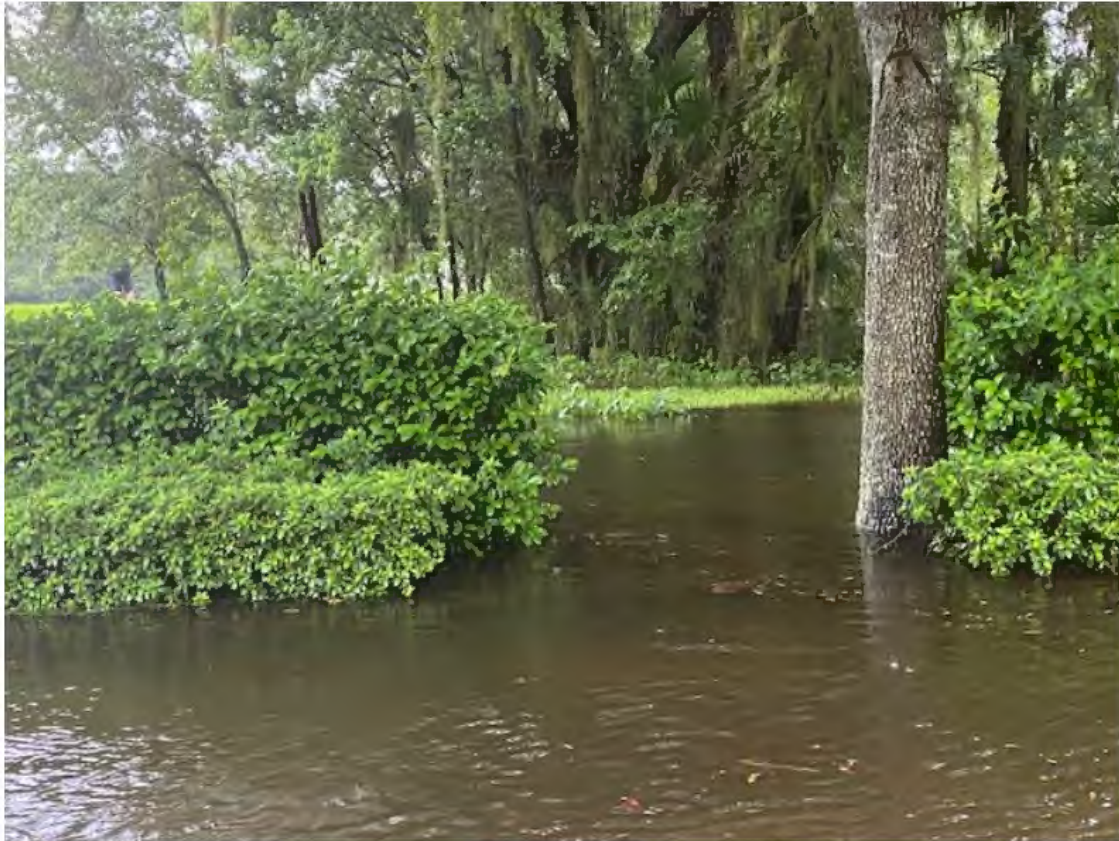
Looking east across Cotillion Blvd from the median island— water flooding street at 8CC Sump, street drain next to tree and storm drains at sump unable to handle the amount of water from rain and outfall from Southern Hills pond. Cotillion Blvd is under about 18" of water at curb.
