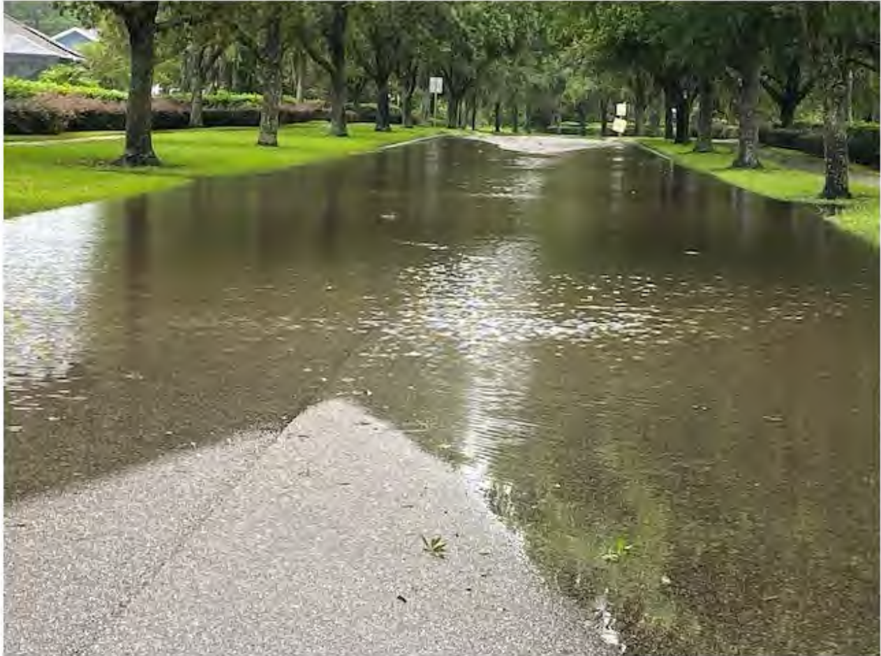
Looking south along Cotillion Blvd, Jennings Trail to Tattnall Way 2nd flooding location – water flooding street. Water was over 12” at deepest point, street drains going into pond 1 (south of sales office) couldn’t handle the amount of water that came down.
