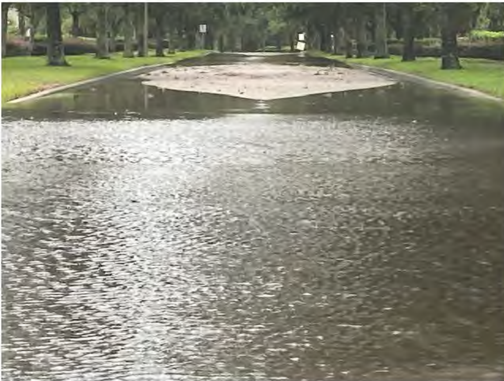
Looking south along Cotillion Blvd, Jennings Trail to Tattnall Way 1 st flooding location – water flooding street was over 12" at deepest point, street drains going into pond 1 (south of sales office) couldn't handle the amount of water that came down.
