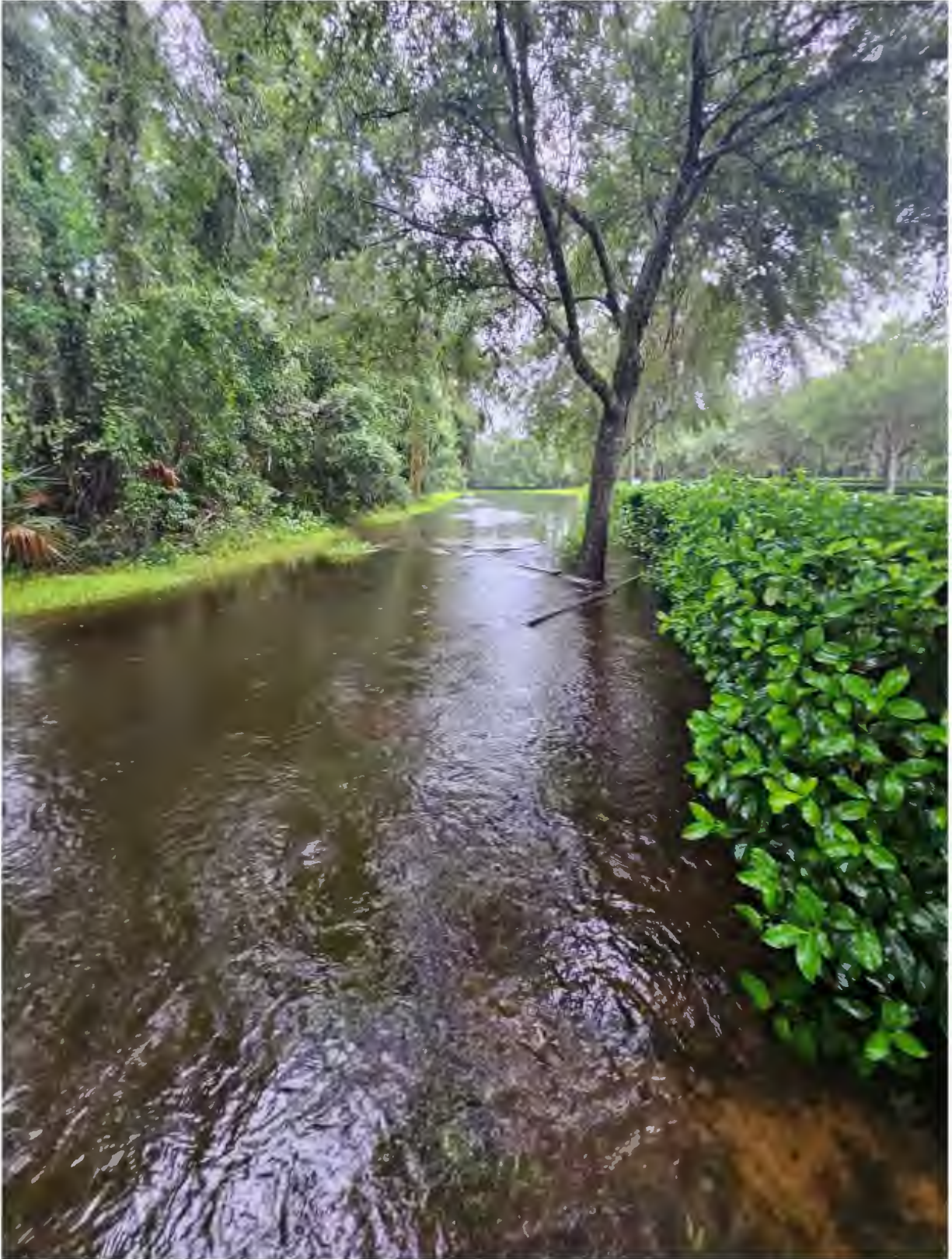
Looking south towards pond 7A – The outfall weir for 7A is just past the tree, Cotillion Blvd is to the right on the other side of the bushes.
