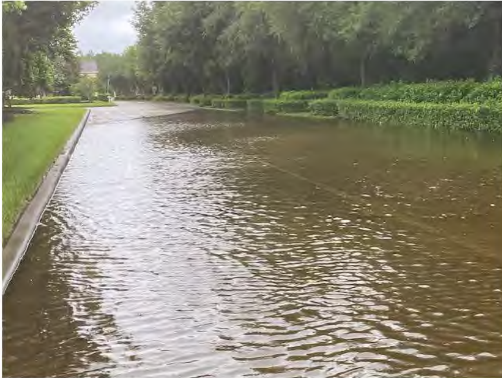
Looking south along Cotillion Blvd entry lane – water flooding street.
